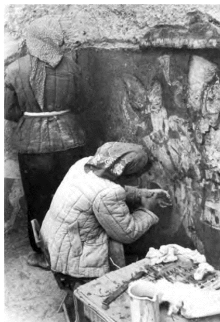
Fig 4. Restorers in process of removing wall painting layer (source: IICAS,2015)
